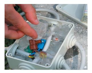
Start filling the void with the gel and press into all areas and corners leaving absolutely no gaps.
