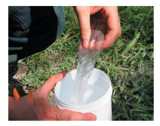
Take the gel out of the tub, equivalent to the size of the void.
