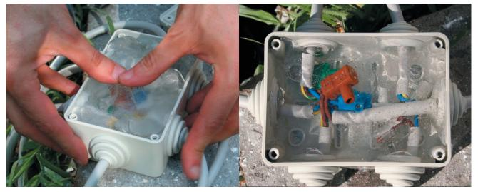
Fill the entire void all the way to the top, ensuring there are no air bubbles or gaps when component is closed. Gel will then smooth out to fill the entire space, so make sure that enough gel is used, if not enough add more.
